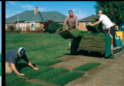
Kesmac Sod Installers carry 4000 lbs. with Specialized Tracks to reduce footprint.
